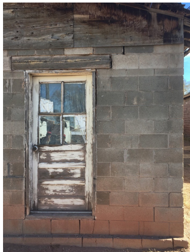
CMU constructed home with visible foundation settlements from exterior corner. Back door no longer operable from wall settlements.
