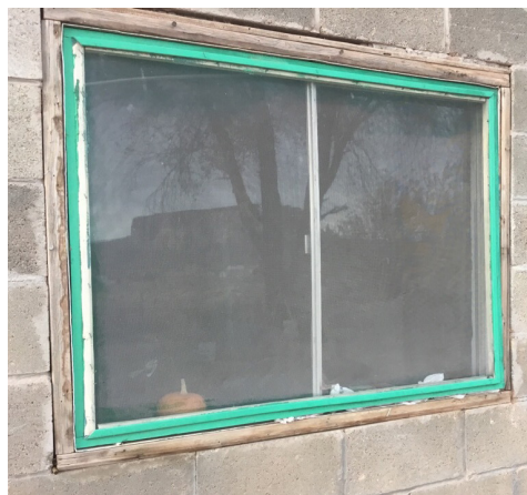
Images of CMU constructed homes with window winterization needed. This unfinished condition provides an opportunity for water infiltration and mold.
