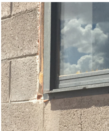
Images of CMU constructed homes with window winterization needed. This unfinished condition provides an opportunity for water infiltration and mold.
