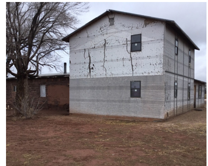
Cement stucco incomplete/ building wrap exposed
