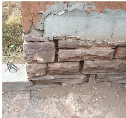
CMU home (partially constructed with stone) with visible foundation settlements from exterior corner.
