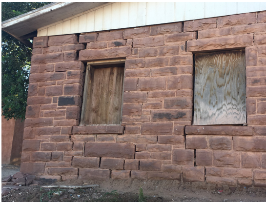
Stone masonry home in Middle Village showing signs of structural settlement. Major cracks (+1/2 inch) visible from exterior.
