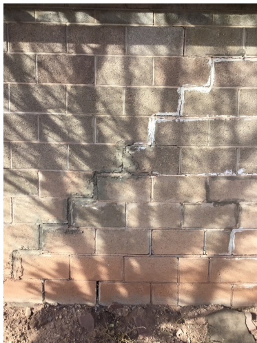
CMU constructed home with visible foundation settlements from exterior. This type of wall patching is common in homes experiencing settlement issues.
