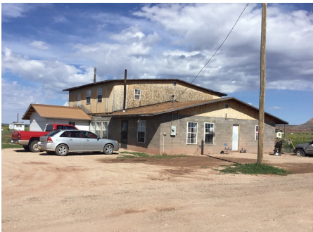
CMU with No finish, OSB/ PWD exposed
